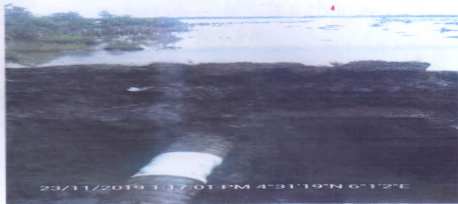
Point patch welded
